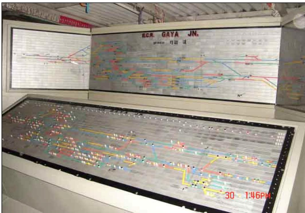
Separate Control Panel & Indication Panel for GAYA Route Relay Interlocking
