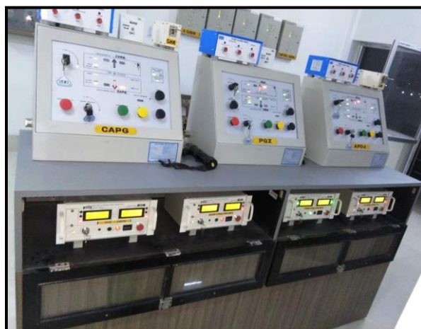
Station Master Room
