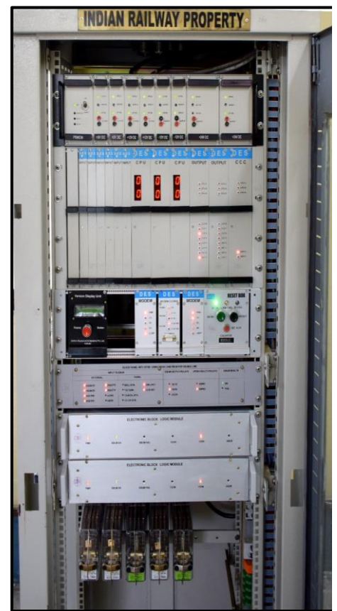
Block Panel with UFSBI (as per IRS: S-105/2012 Ver.0) with Dual EBLM
